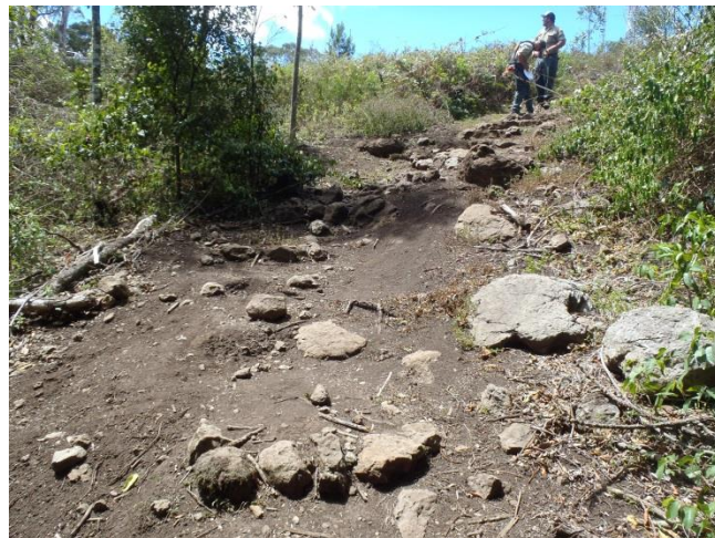
Working on the Russell Park walking track
